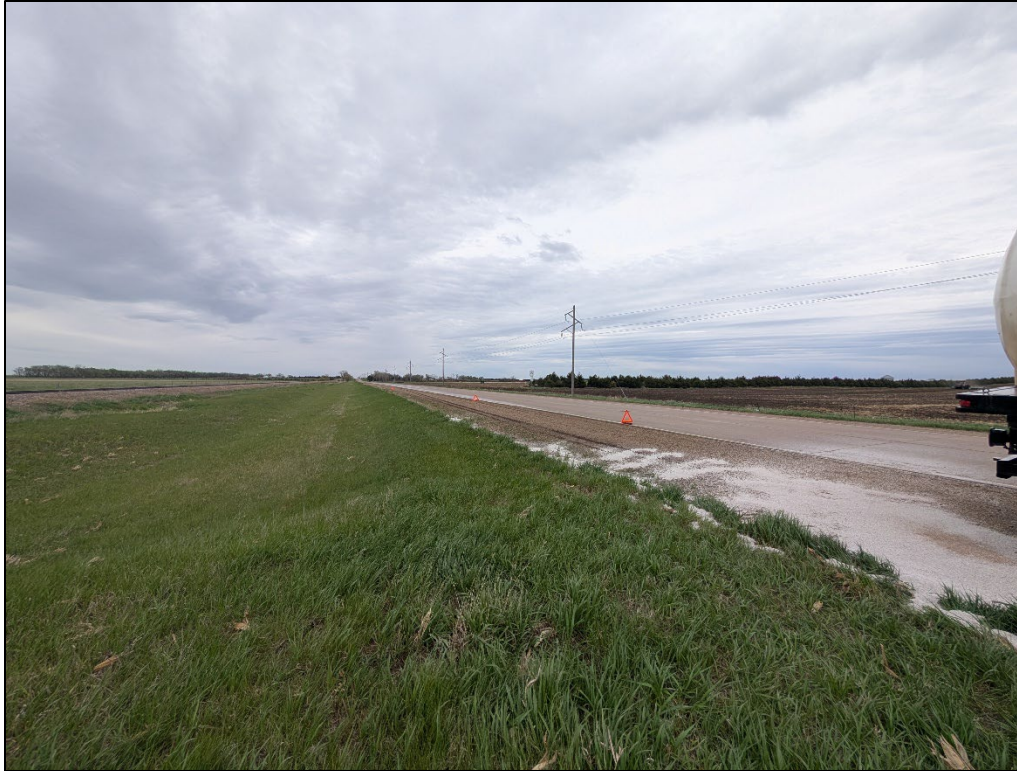
05-04-2026 Impacted Shoulder And Roadway West Of Truck And Tank
