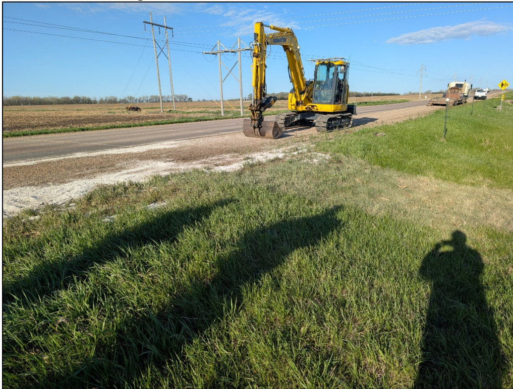
05-08-2026 Prior To Excavation
