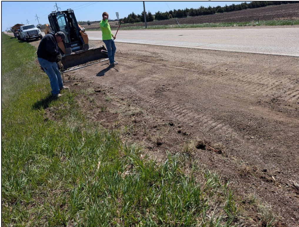
05-08-2026 Post Shoulder Scrape Manual Touch Up Work
