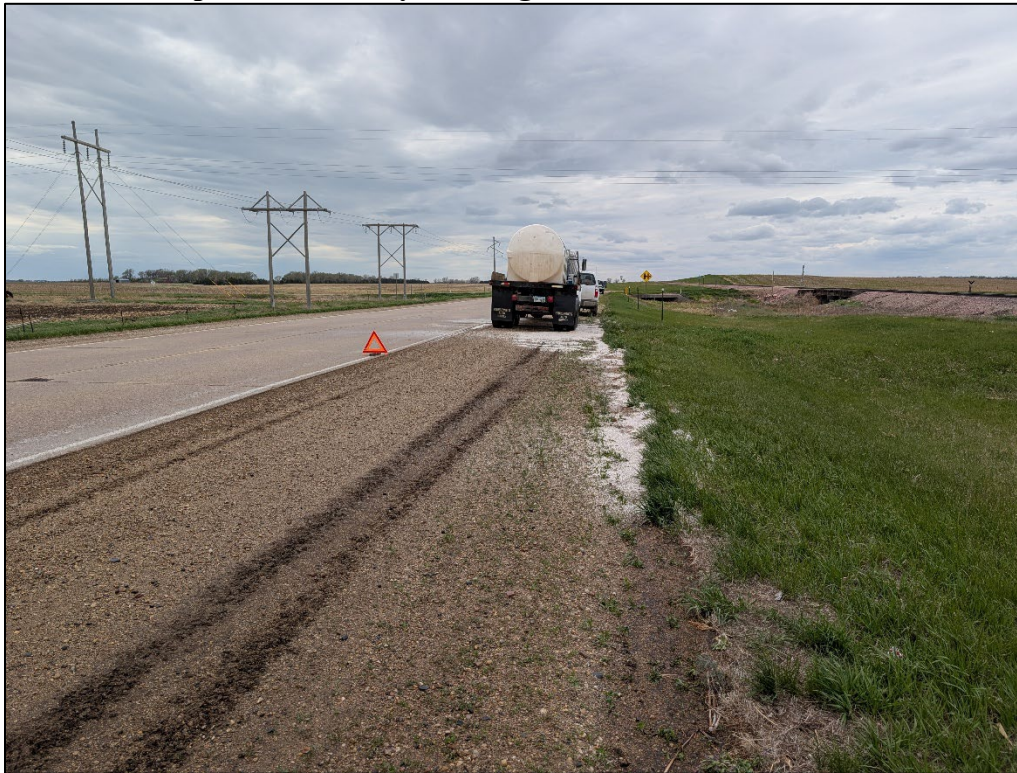
05-04-2026 Truck View From East
