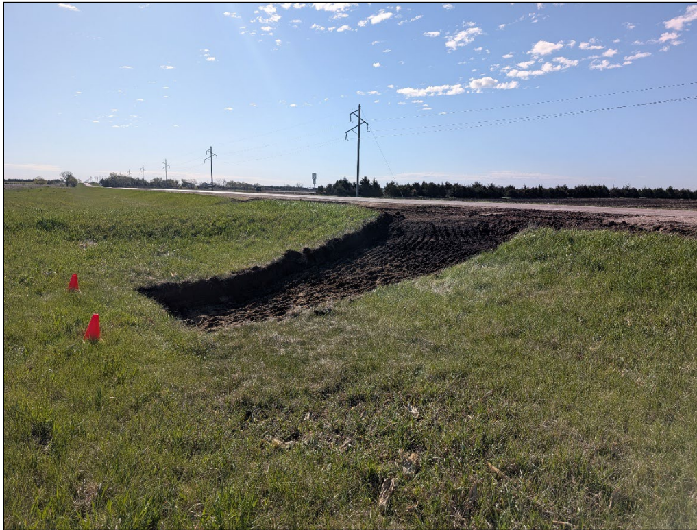
05-08-2026 Post Excavation Awaiting Backfill
