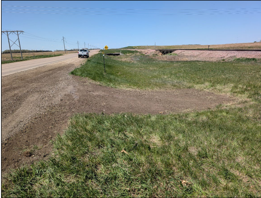
05-08-2026 Excavation Backfilled And Shoulder Scraped
