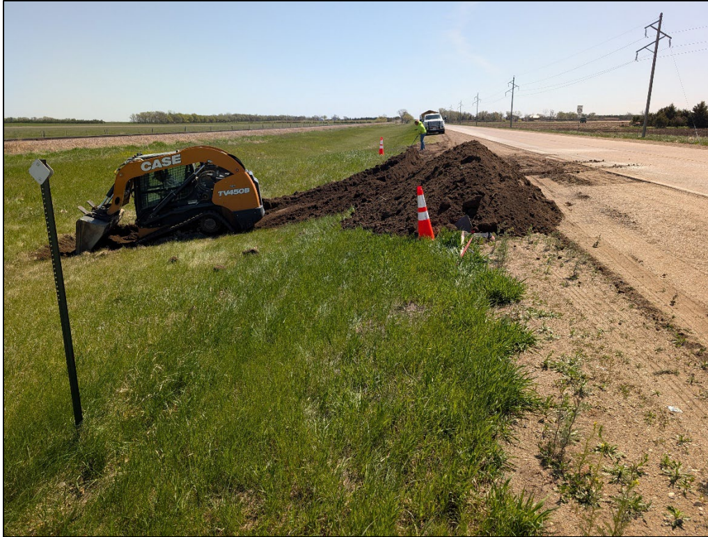
05-08-2026 Backfilling
