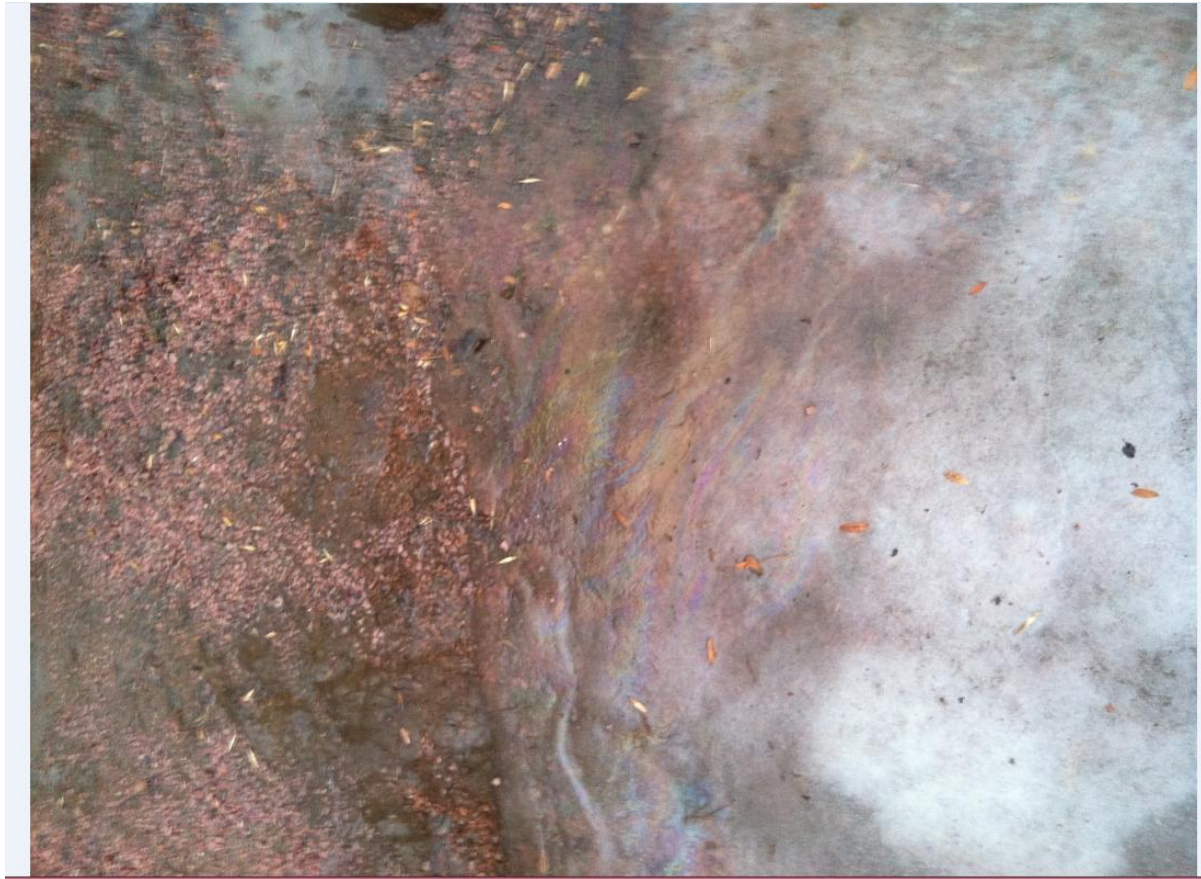
Photo #4: Water pumped from basement to driveway with signs of fuel oil.
