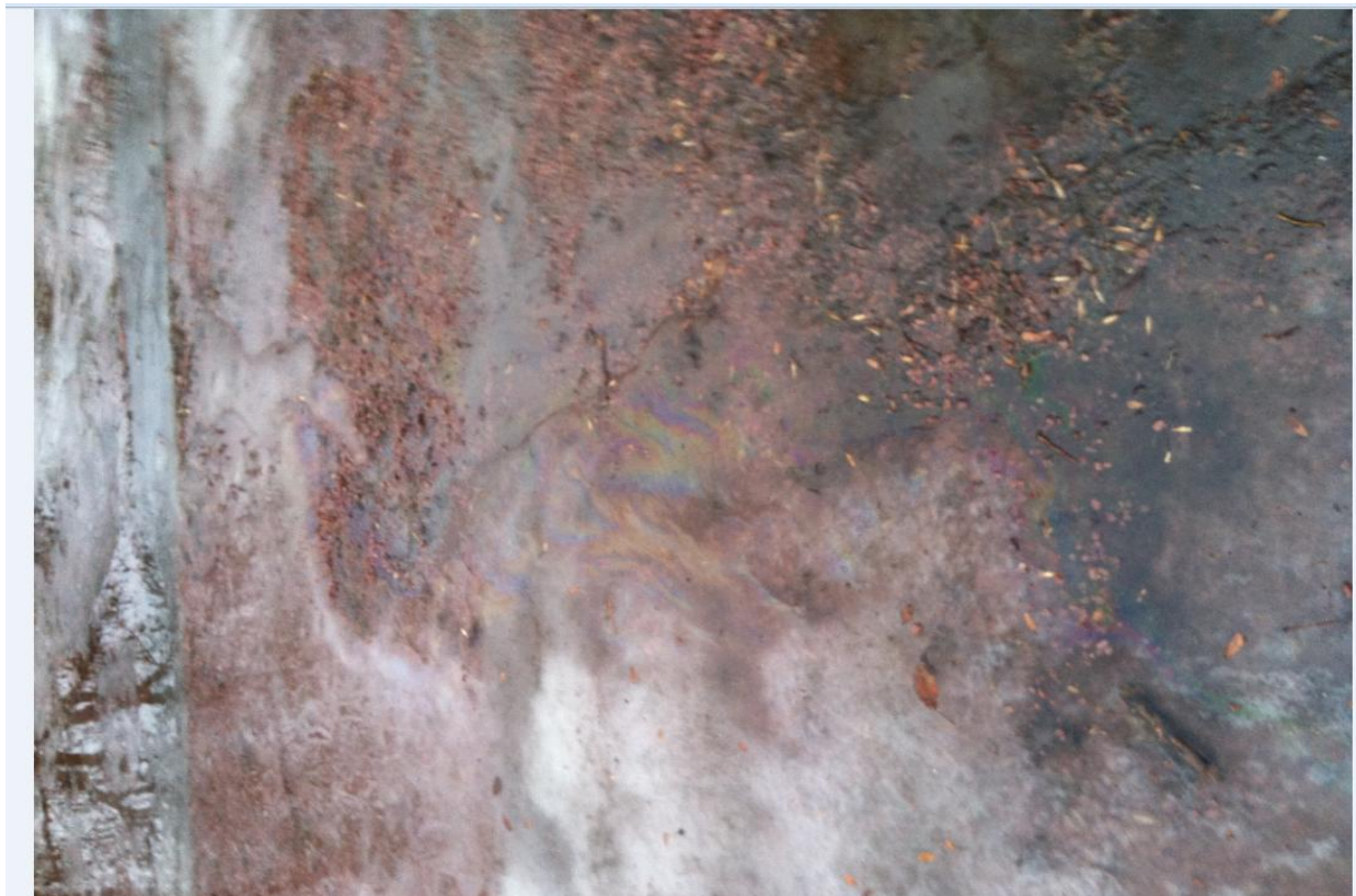
Photo #3: Water pumped from basement to driveway with signs of fuel oil.
