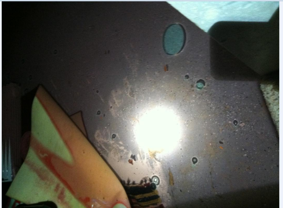
Photo #5: 8" water in basement with spots of fuel oil.
