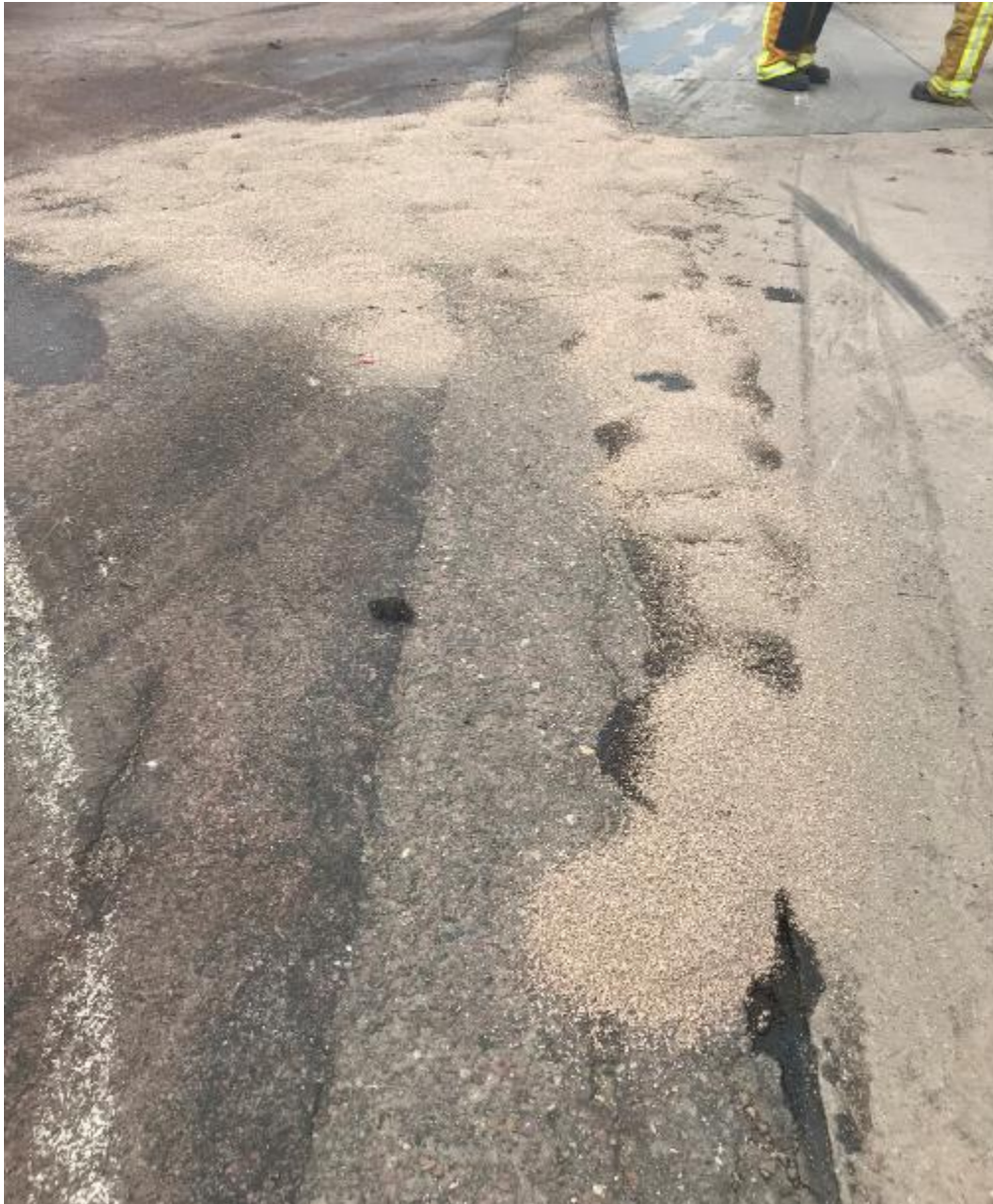
Photo #: 9-Engine oil covered with floor dry
