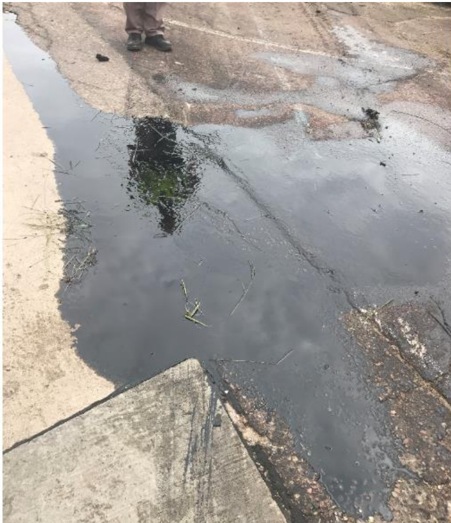
Photo #: 8-Engine oil, leaked on HWY when semi-tractor was pulled from the ditch
