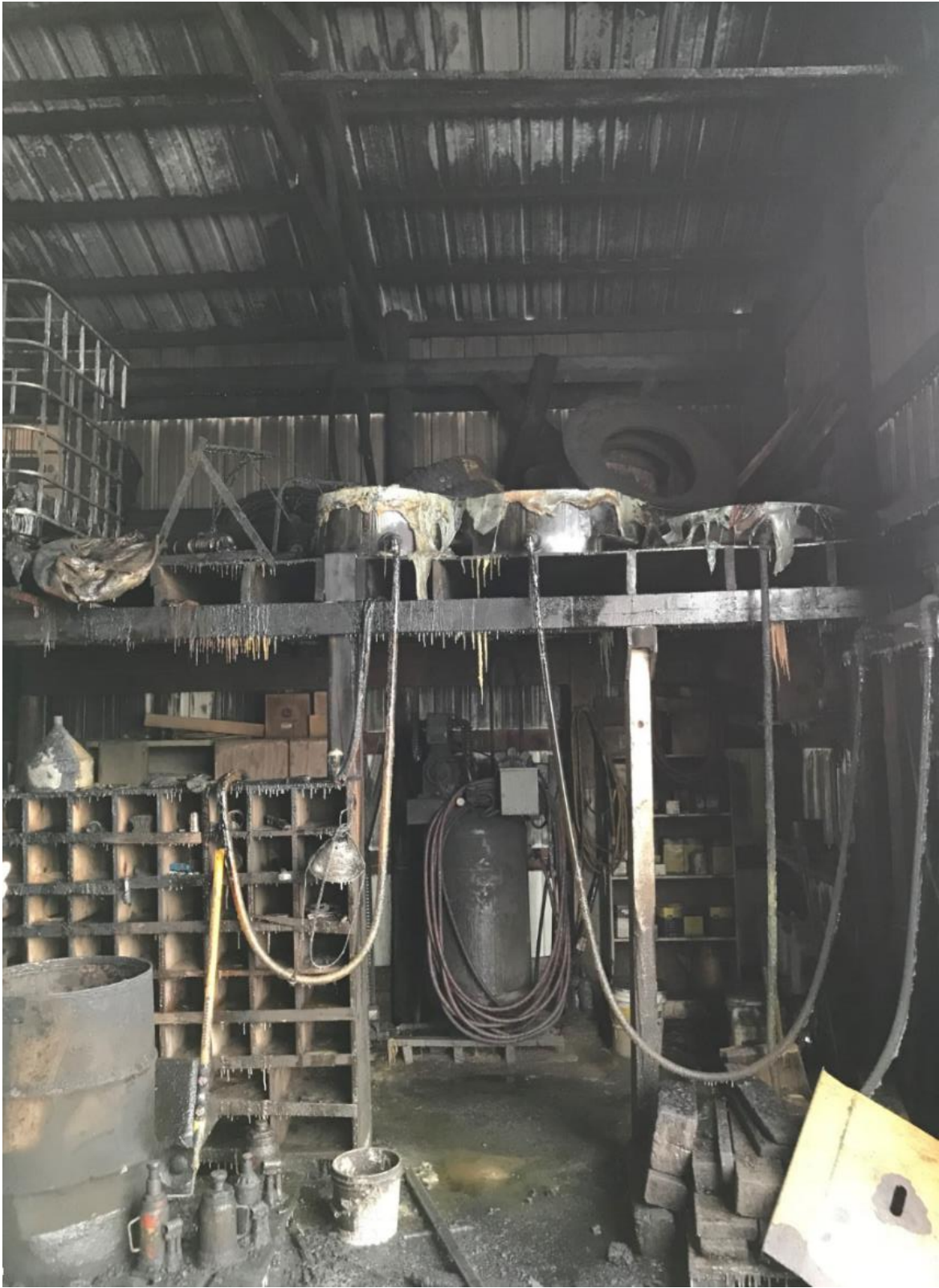
Photo #: 3-Shop and Fire Area
