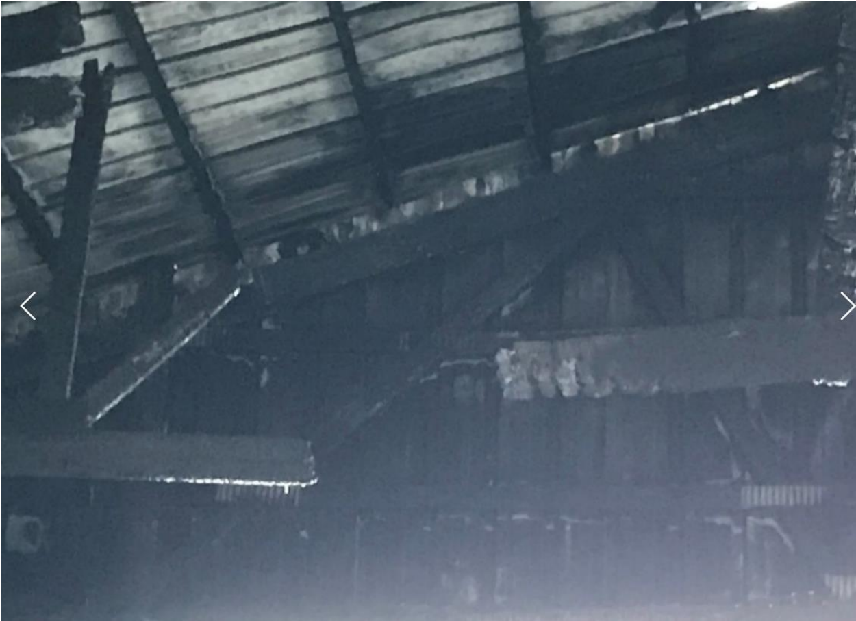
Photo #: 8-Trusses Damaged2
