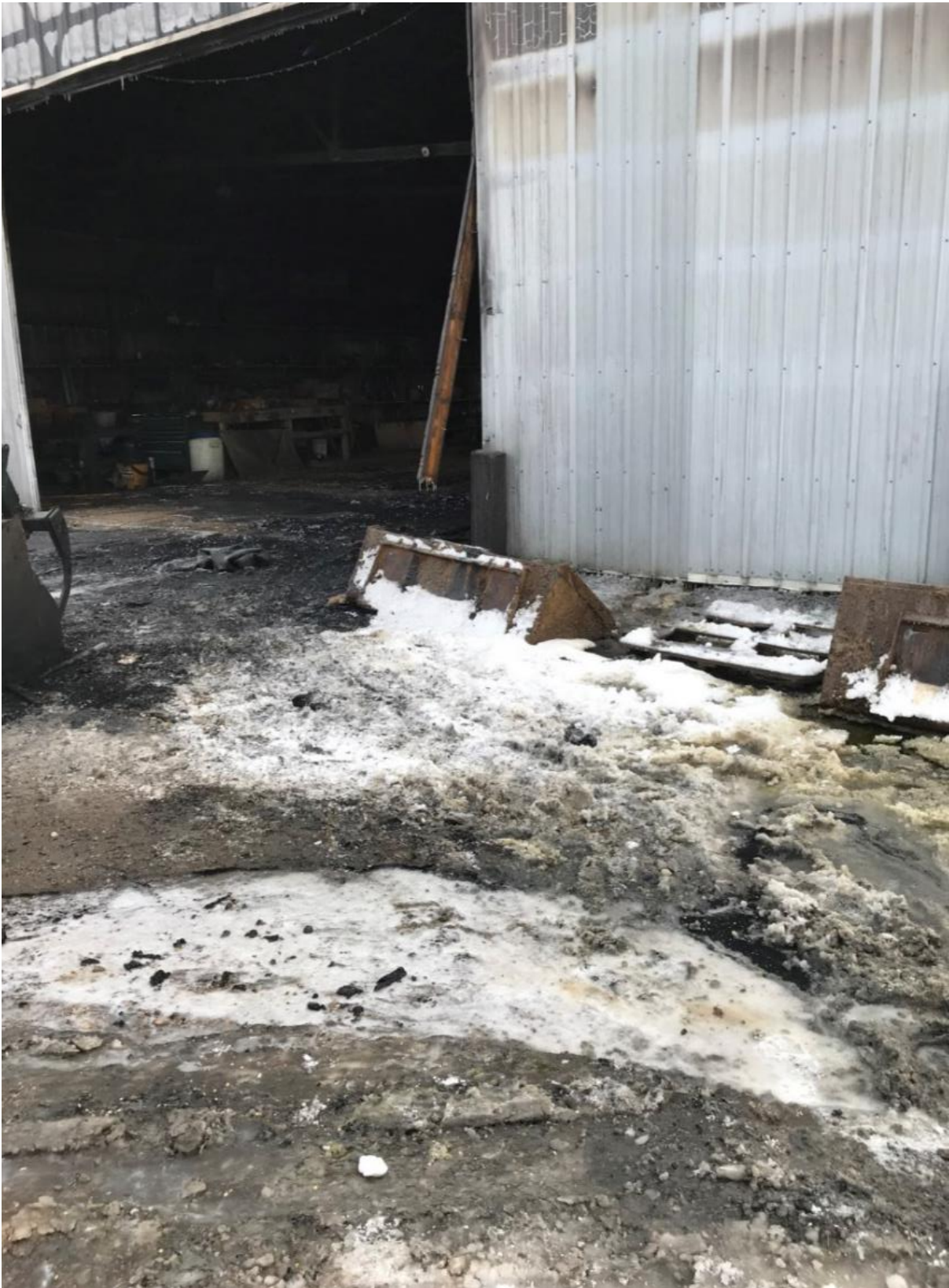
Photo #: 9-Shed-West Side
