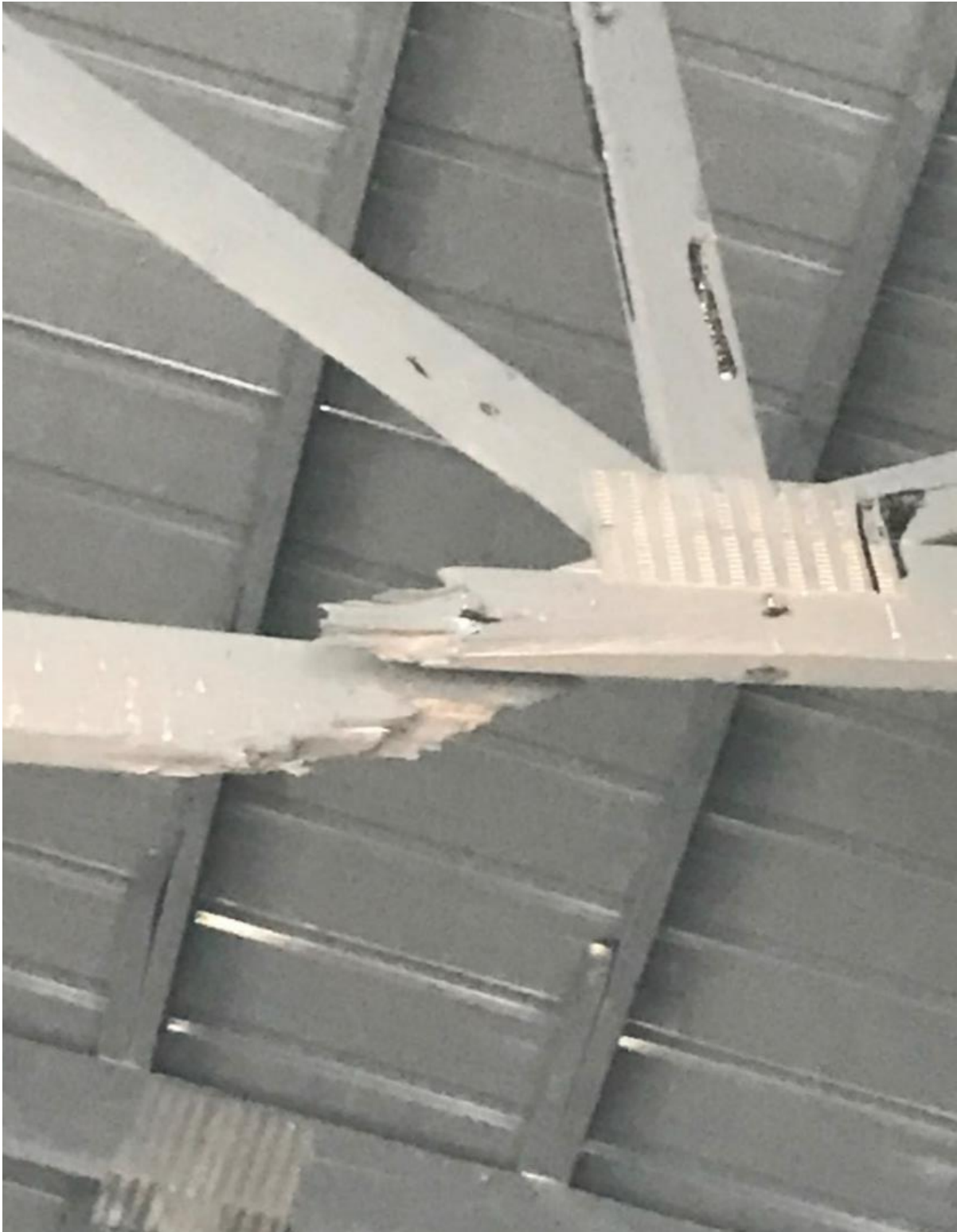
Photo #: 7-Trusses Damaged
