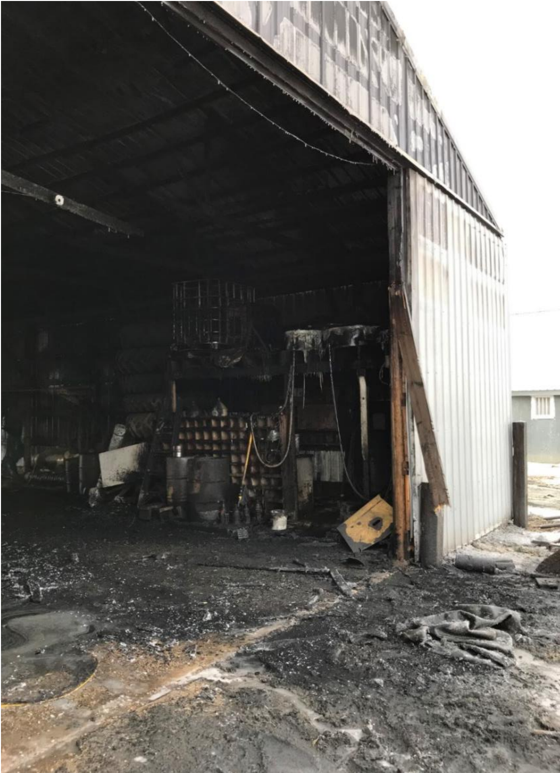
Photo #: 2-Shed-West Side and Fire Area
