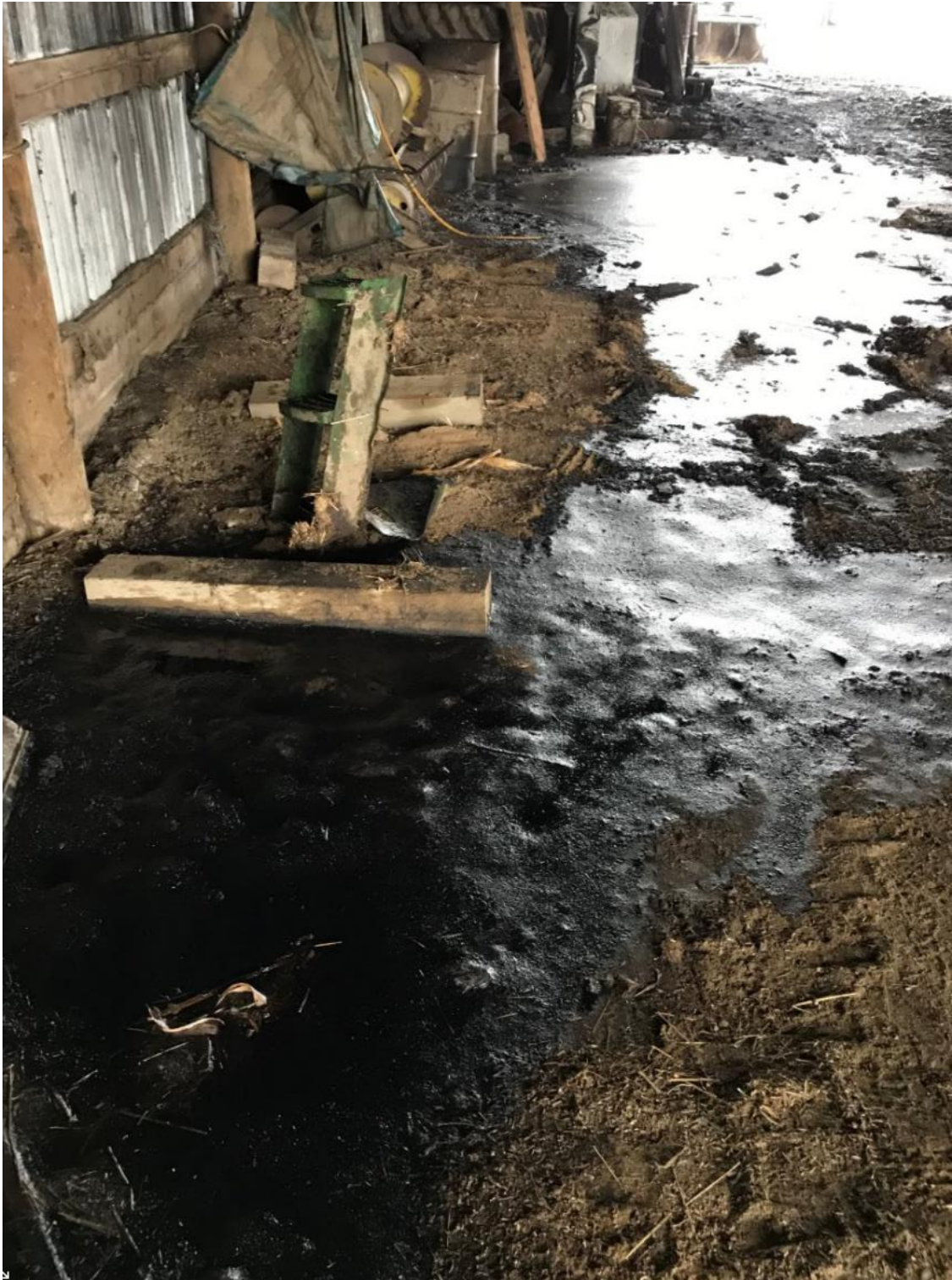
Photo #: 5-Shop Floor with Oil Pool
