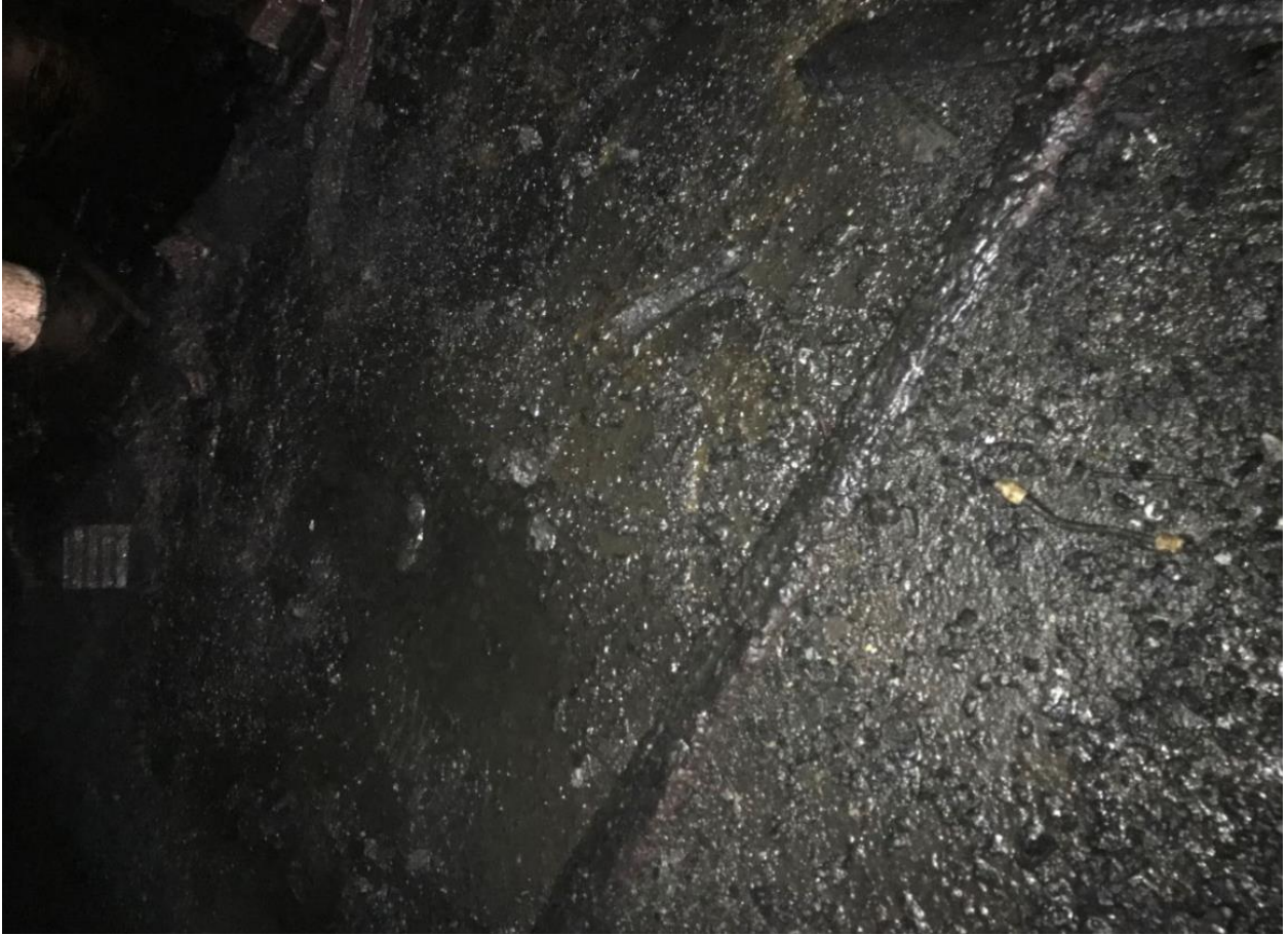
Photo #: 6-Shop Floor-Oil Saturation
