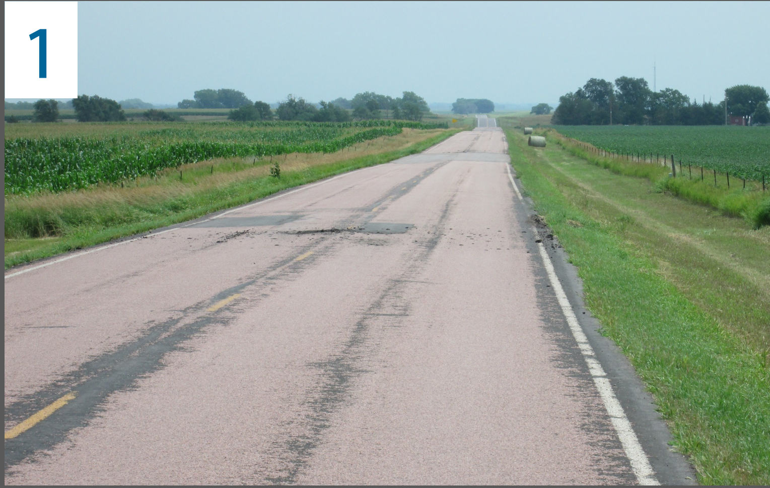
Pavement deterioration along 265 th Street.
