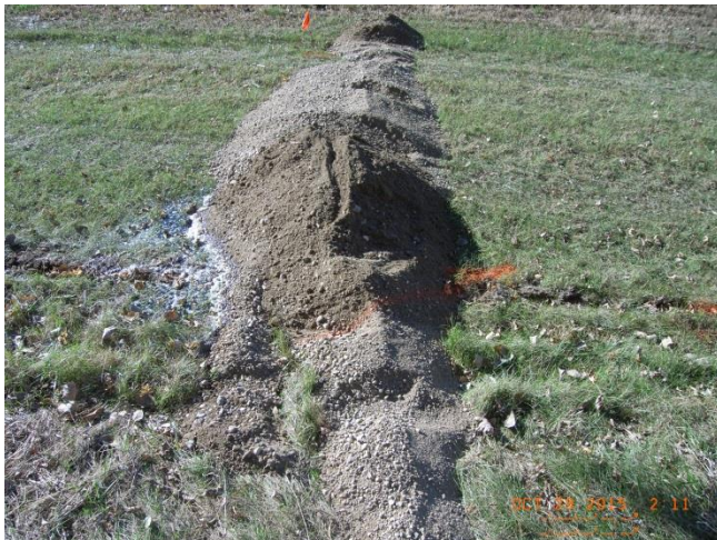
This picture was taken facing west, showing one of the dirt dikes that were built to contain the spill in the east ditch.
